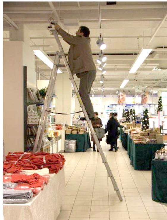
**Picture:** The ladders in the picture on the left do not comply with safety regulations in the workplace anywhere in the world. Minimise personal injury by using only suitable ladders and stands. The ladder in the right side picture is a better choice compared to the ladder in the previous picture, but still is not necessarily the best option. With long ladders two people should be present, one to secure the ladder and hand over or take tools and supplies, the other on the ladder.
